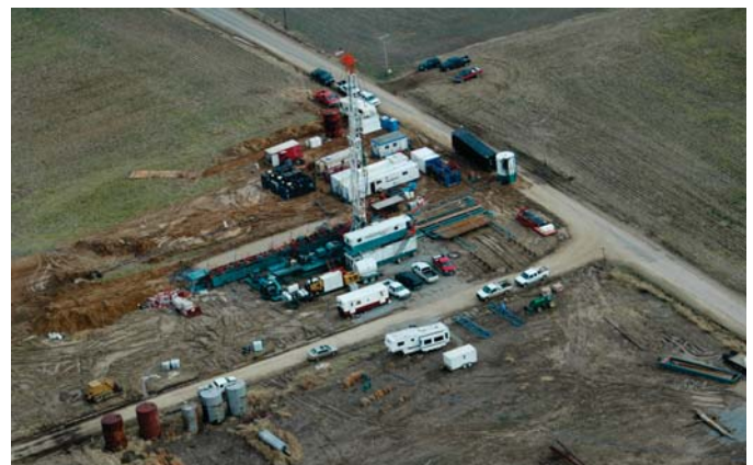
FIGURE 3 MPD Surface Equipment Setup (Well No. 2)
